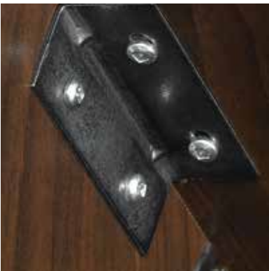
Tamper Proof Screws on All Exposed Connections
